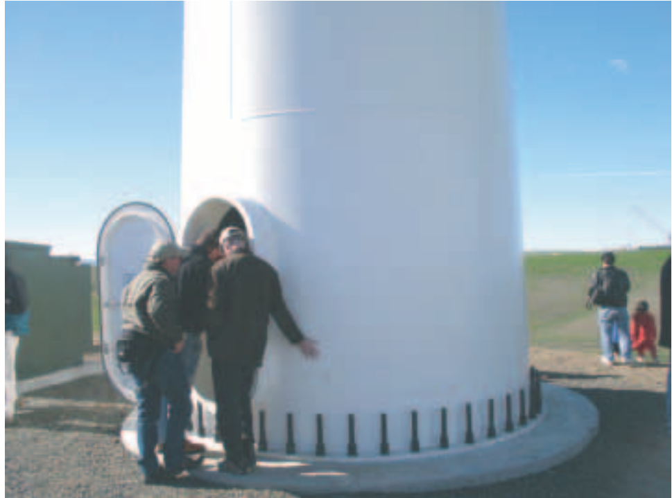
FIGURE 1.24. Entering the maintenance hatch in one of the Solano wind turbine towers. Courtesy of D. K. Lieu
