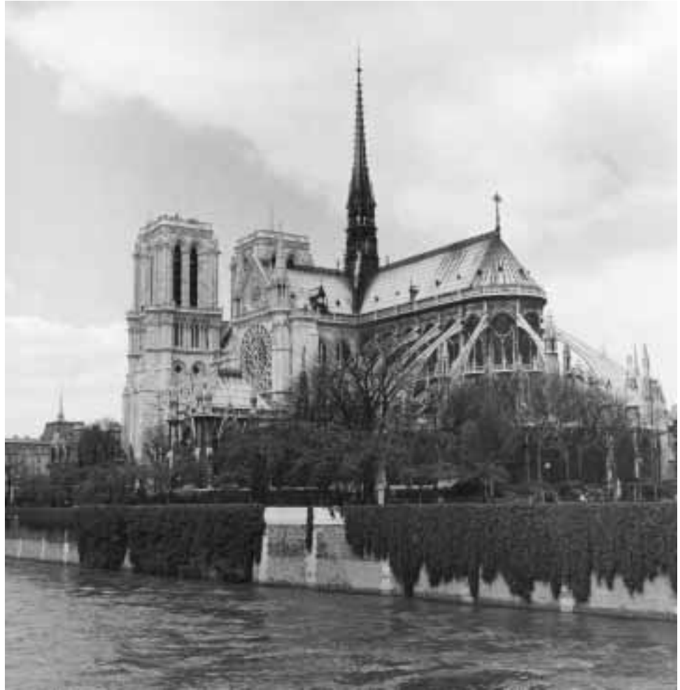
FIGURE 1.06. Flying buttress construction used to support the exterior walls of Notre Dame Cathedral in Paris. Courtesy of Getty Images
